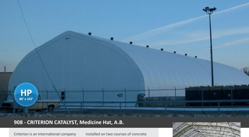
Criterion is an international company that supplies catalysts, process technologies and catalyst services for a wide range of refining applications. An 80' wide model HP MegaDome, was installed on two courses of concrete Lock-Blocks, on an existing asphalt paved slab. To compensate for the slope of the existing pavement customized base adjusters were installed.
